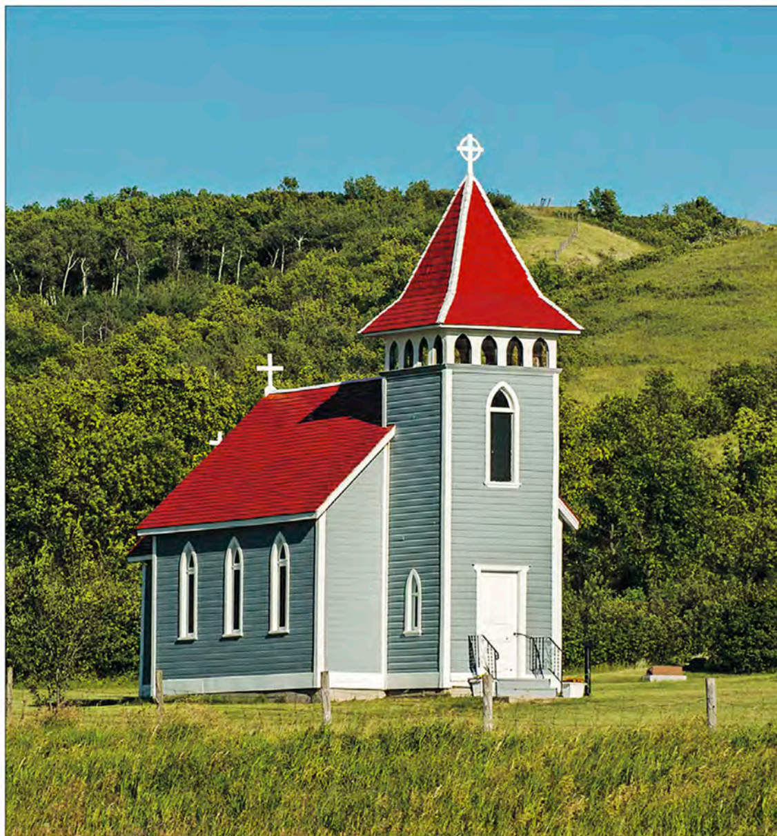
There are lot of old churches to see in the valley, including the Kennel Church.
